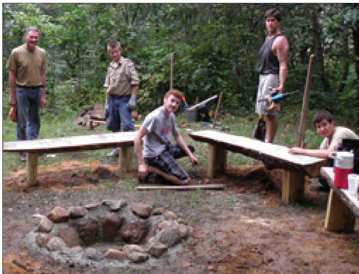
Dodgeville Eagle Scout, Gus Quade, and helpers work on the new benches and firepit at Friendship Center.
